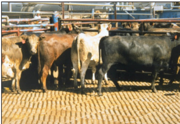
A good sample of non-slip flooring.
